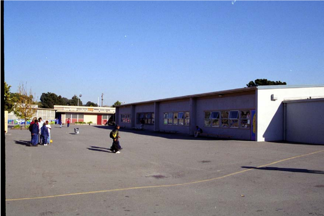
Figure 7: Main Classroom Building, north face
