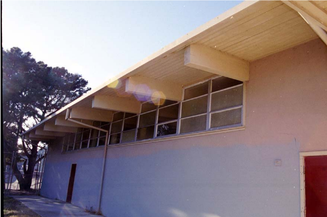
Figure 4: Multipurpose Building, south face
