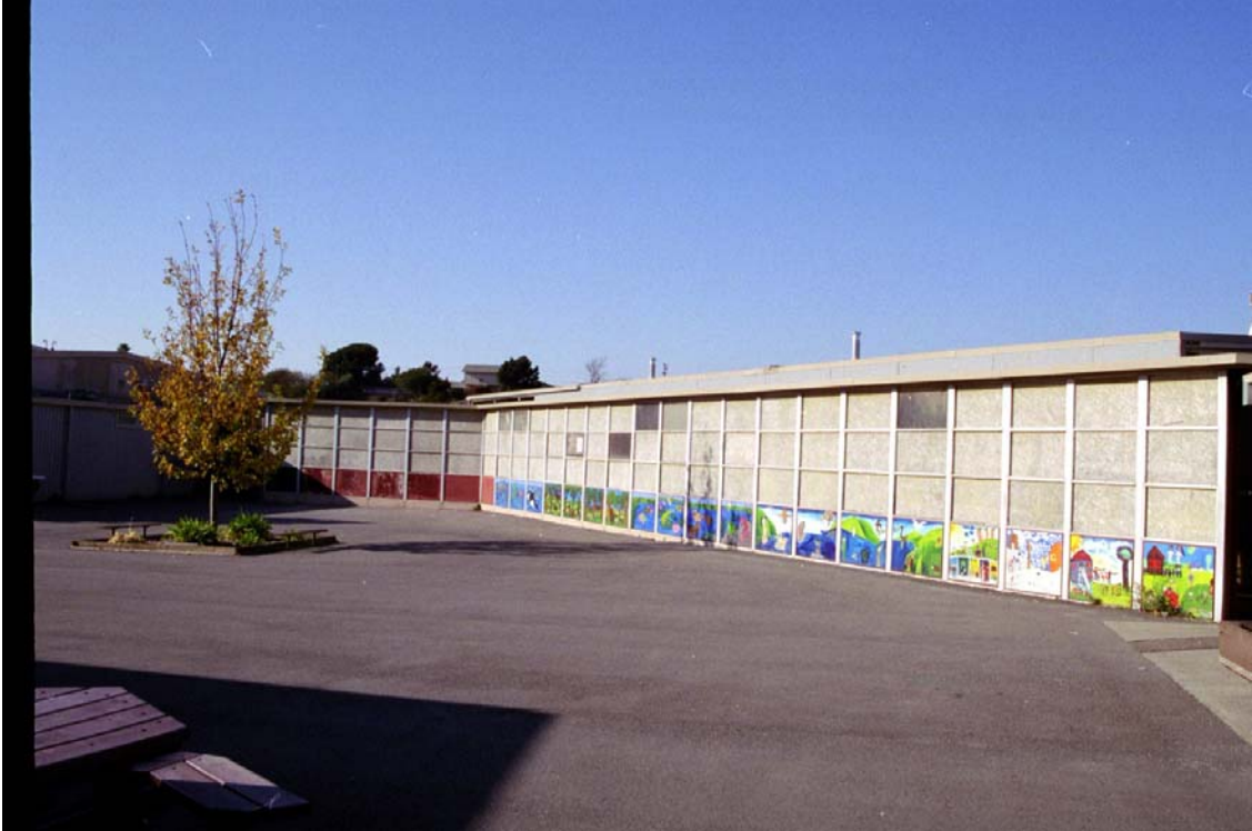
Figure 9: Covered Walkway, outside
