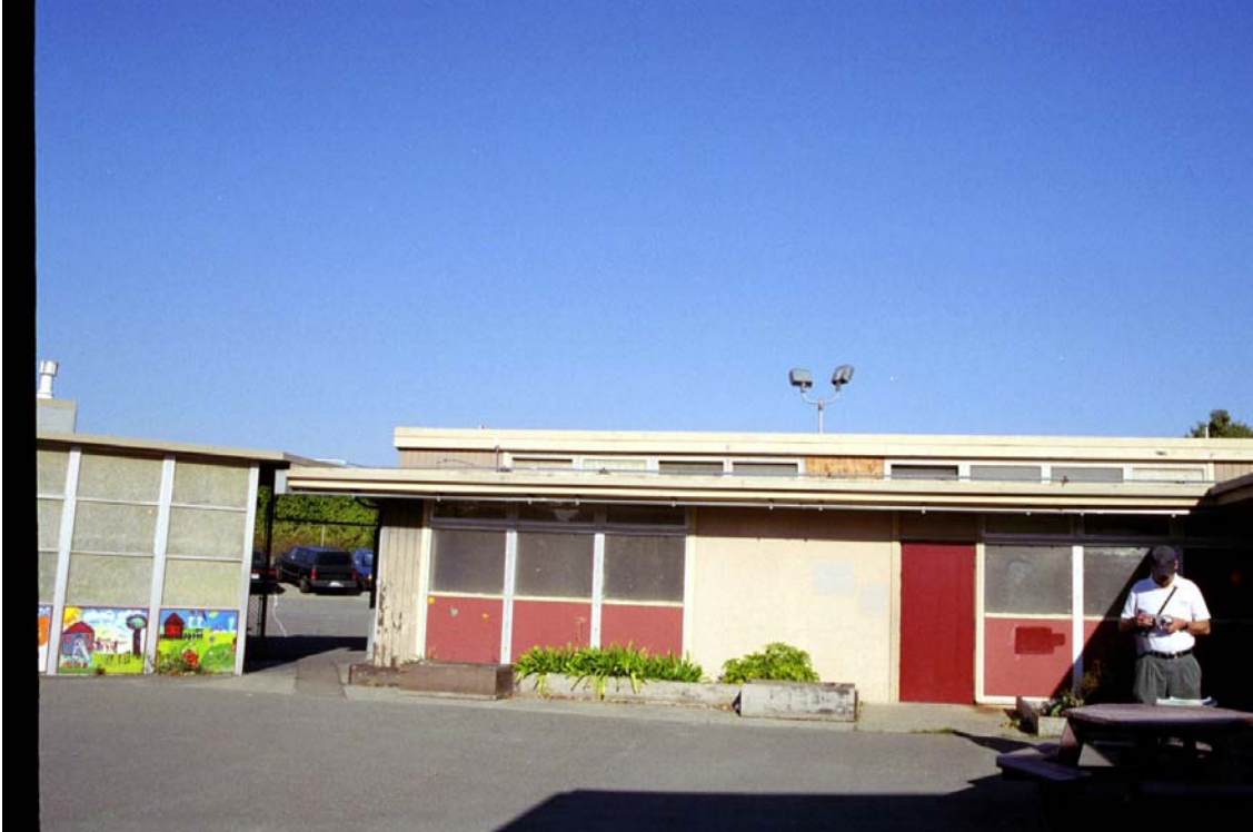
Figure 8: Main Classroom Building, north wing
