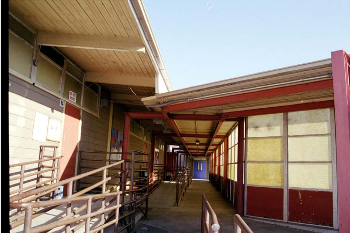
Figure 10: Covered Walkway, inside
