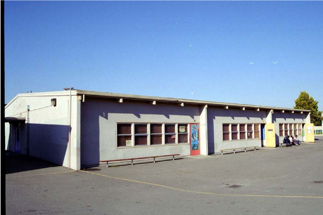
Figure 11: Classroom Building, south face
